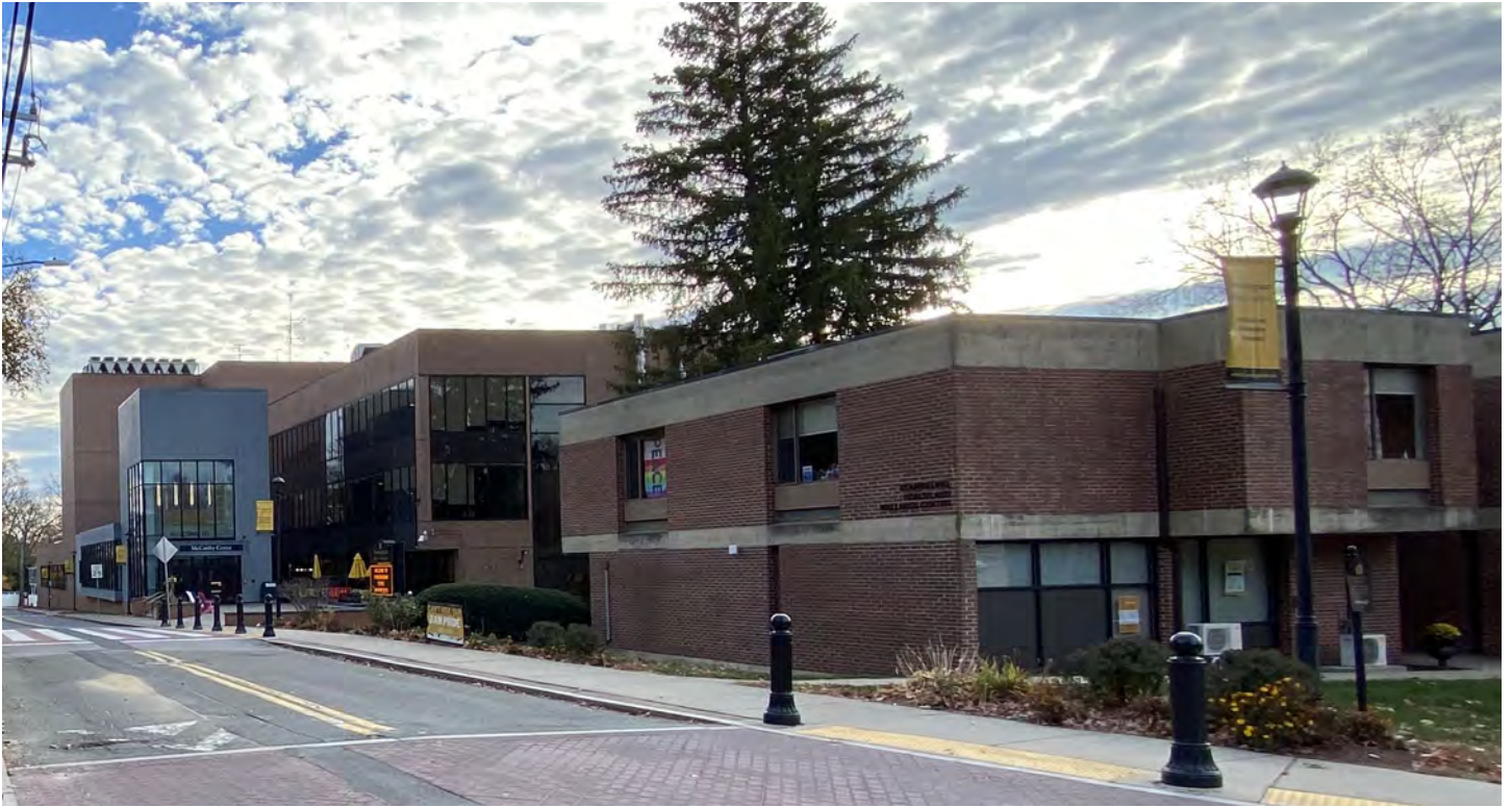
Existing View of Foster Hall from State Street
